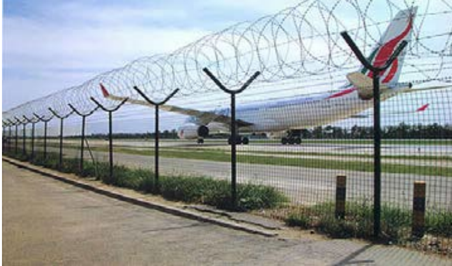
Figure 2. Well-maintained fence, at least 3m high, no gap at the bottom and dig protection are required.
