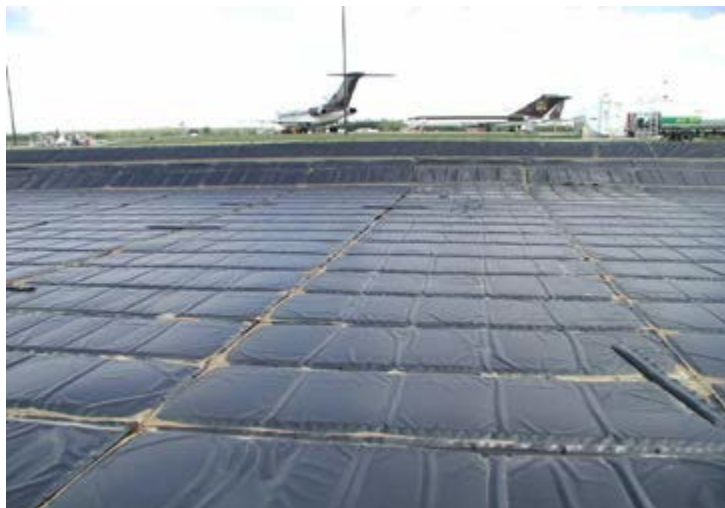
Figure 5. Permeable floating cover at sewage
