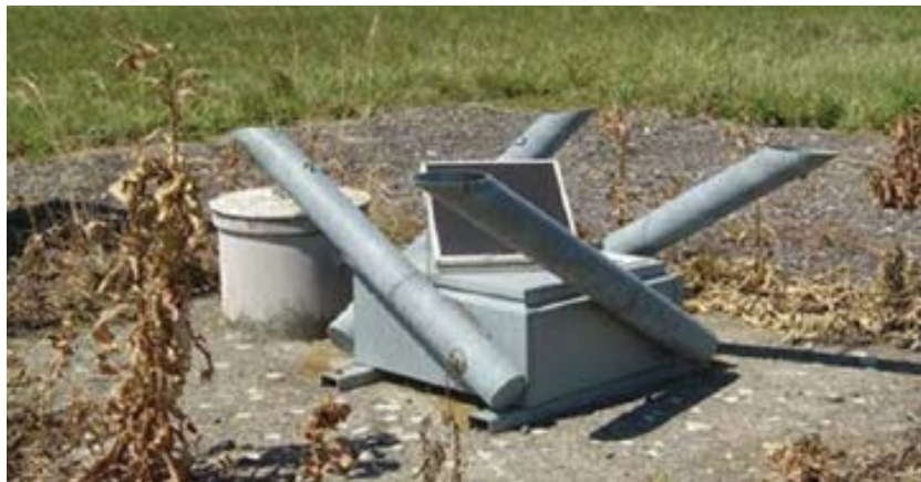
Figure 10. An underground stationary gas-powered noise generator
