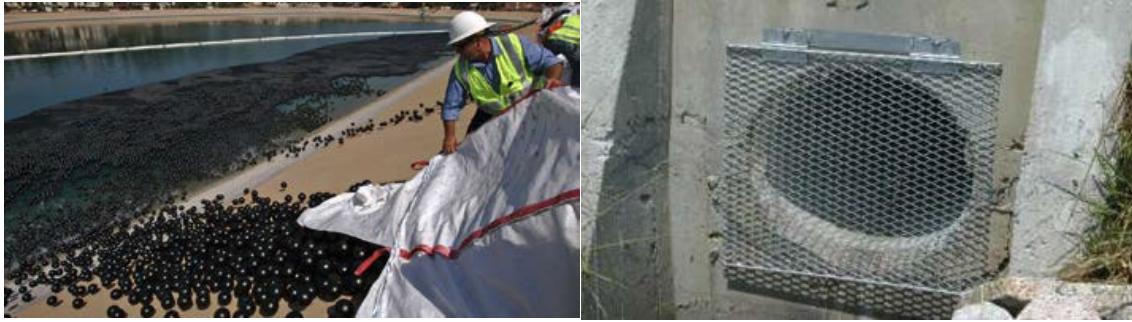
Figure 1. Floating balls and bird netting to cover the water, and drainage opening protection
